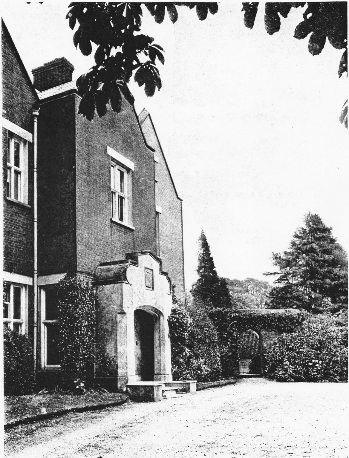
Entrance Porch, South-West.
